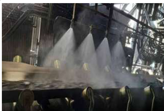
Fig.4: Mechanically Actuated dust suppression system on the conveyors of CHP
