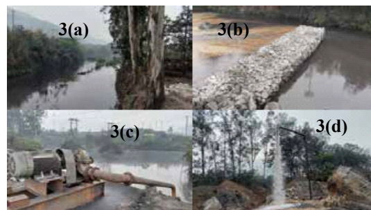
Fig.3(a) Creation of water body; 3(b) Gabion wall for silt control; 3(c) Installation of Pump; 3(d) Tanker filling system.
