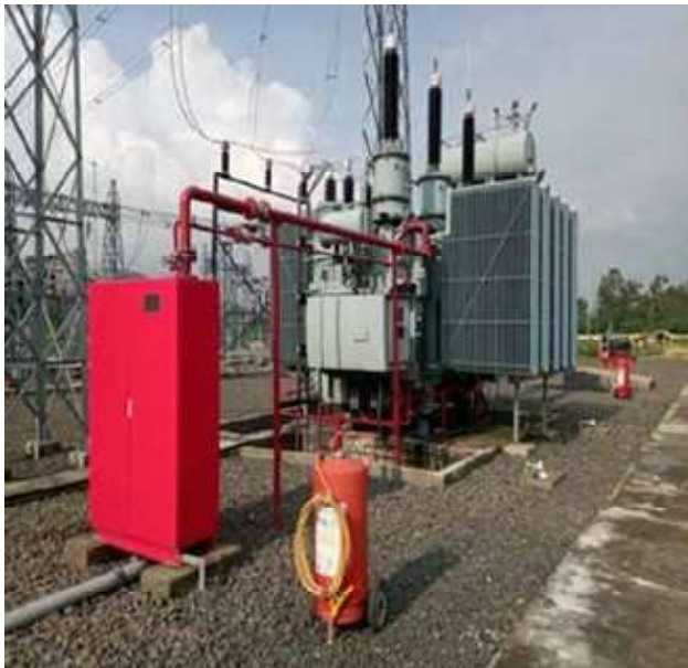
Fig.1: NIFPS in transformer
