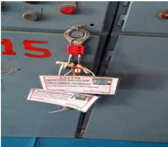
Fig.2: Lockout arrangement
